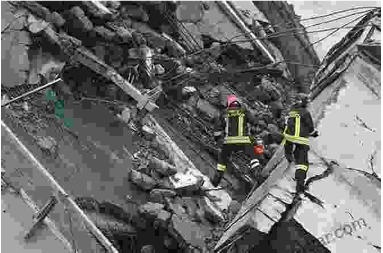
The Morandi Bridge collapsed on August 14, 2018, killing 43 people.
